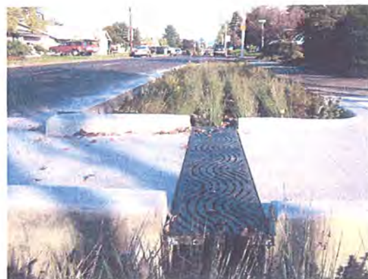
Figure 2-23: A trench drain connects runoff between two landscape areas.
