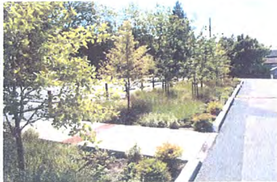
Figure 2-70: A large rain garden retrofitted in a school parking lot.
