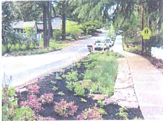
Figure 2-52: Residential street with a vegetated swale.
