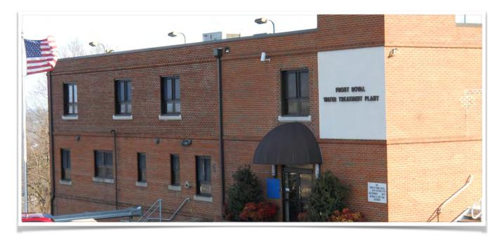
quality and achieve compliance with recent treatment requirements. The work includes the installation of ultra-violet treatment systems at the plant, additional chemical feed improvements, additional aeration improvements at storage tanks, and other enhancements. The project award was for \$2,684,000 and is anticipated to be completed by October 2015.
